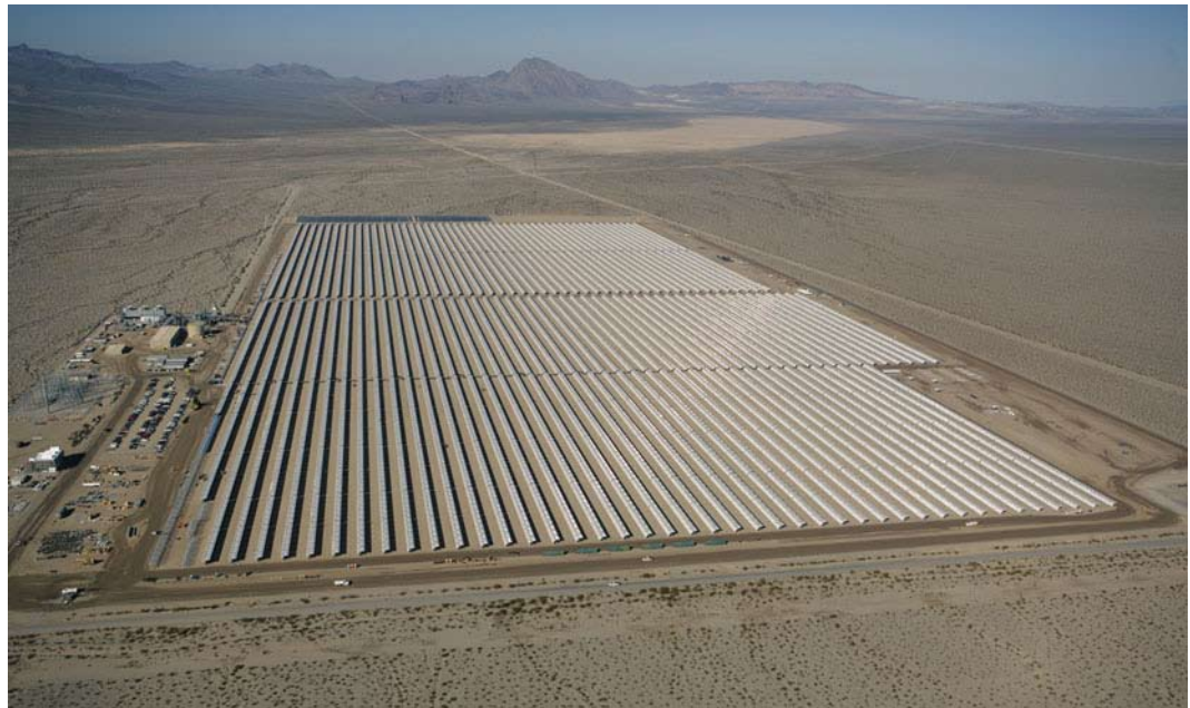
Photo: The Nevada Solar One Power Plant (64 MW) in Nevada, USA Photo: Acciona Solar Power Inc.
