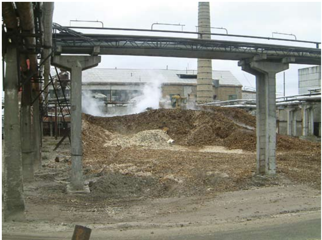
The Zheshart gas to biomass fuel switch project in the Komi Republic, Russia; Source: TGF
