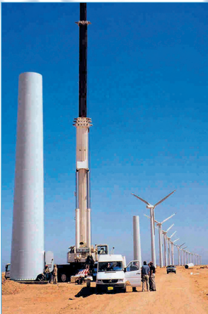
Constructing the Zaafarana wind farm, Egypt
